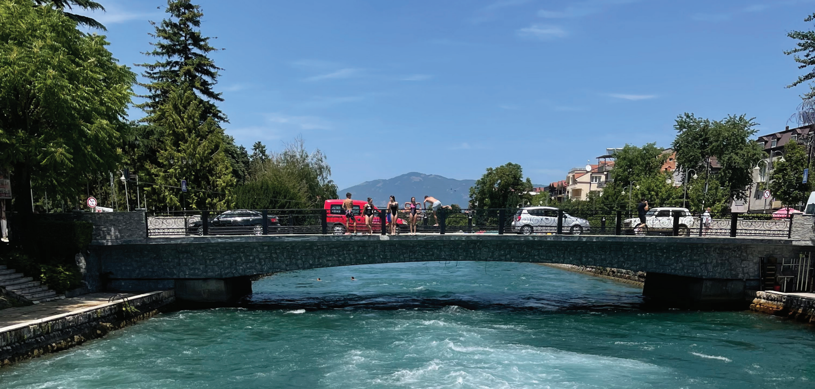
Removing deposited sediment and overgrown vegetation from the river led to resilient flood risk planning in the Black Drin River, Struga, North Macedonia Photo by UNDP Euroasia
